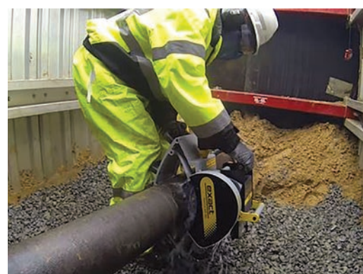
Cutting pipes in the trench
